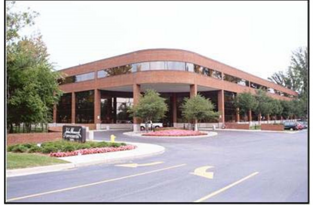
John Hancock 32000 Greenfield, Dearborn (80,000 square feet)
